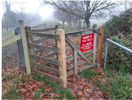
Repaired hanging post on Kissing Gate (west) close to Badgers Crossing
