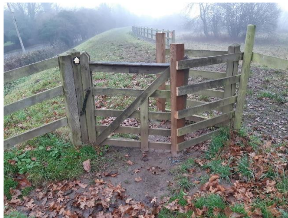
Replacement post on Kissing Gate (east) close to Badgers Crossing
